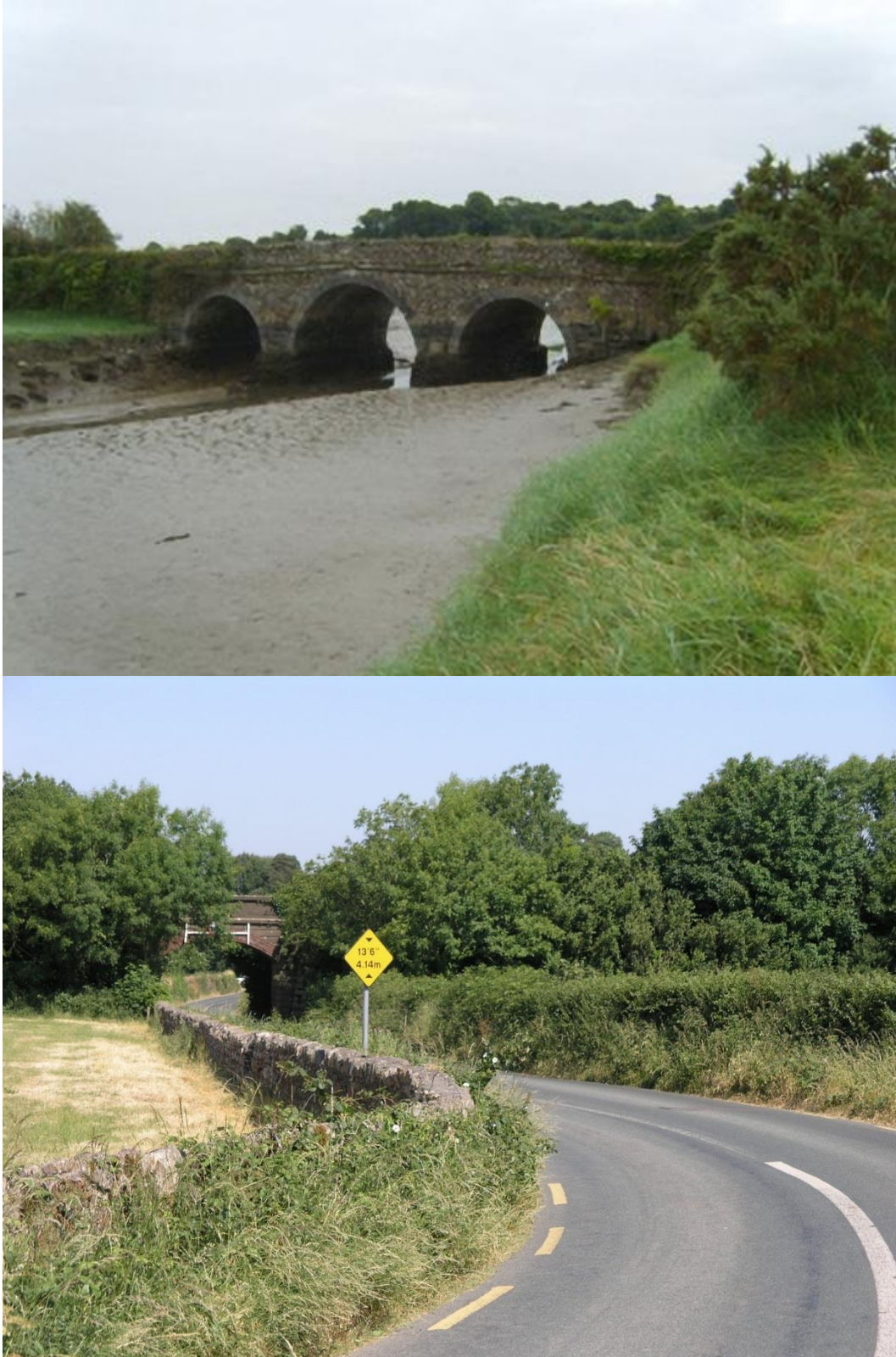
Figure 10.22: Dunbrody Bridge and Railway Bridge
