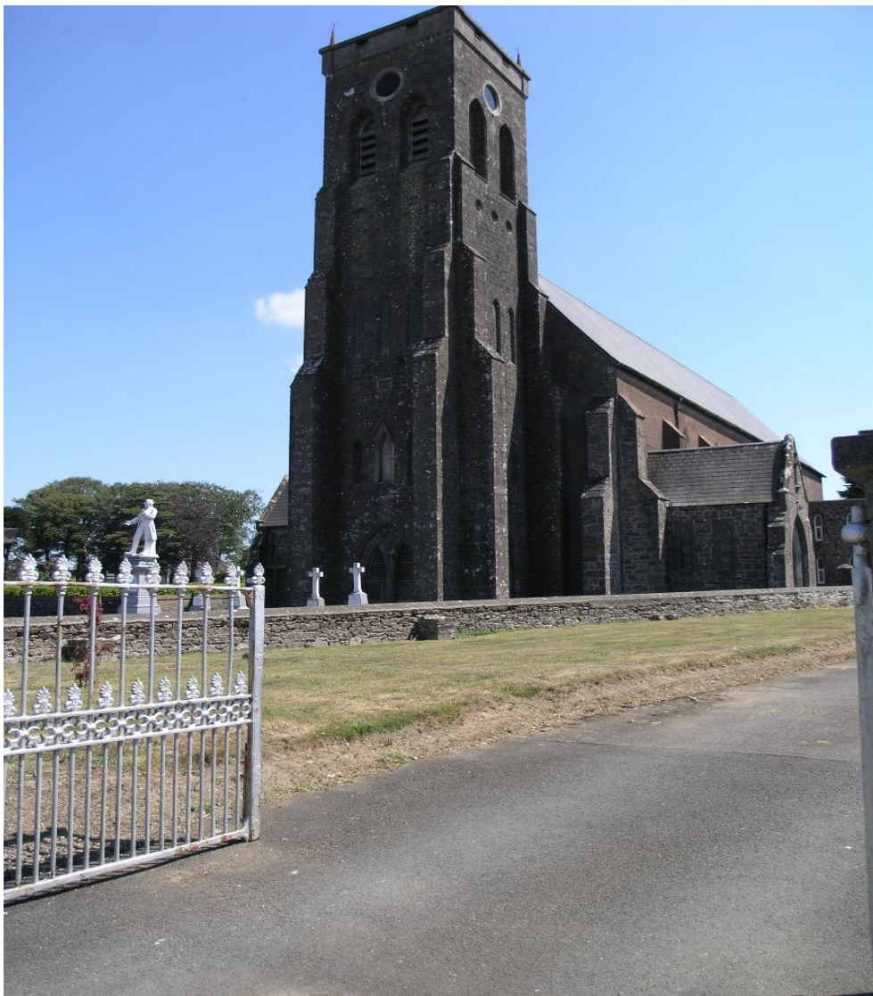
Figure 10.20: Pugin-designed church at Ramsgrange
